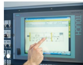
Individually programmable control
